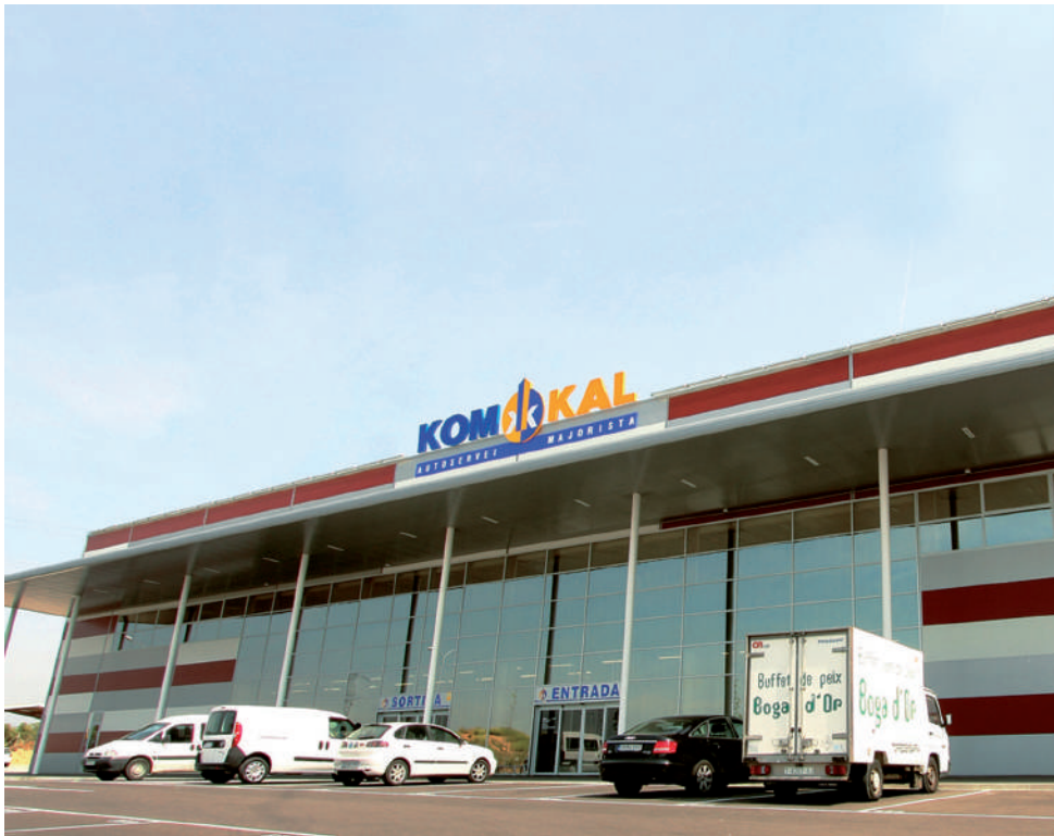
Komkal Industrial Building
